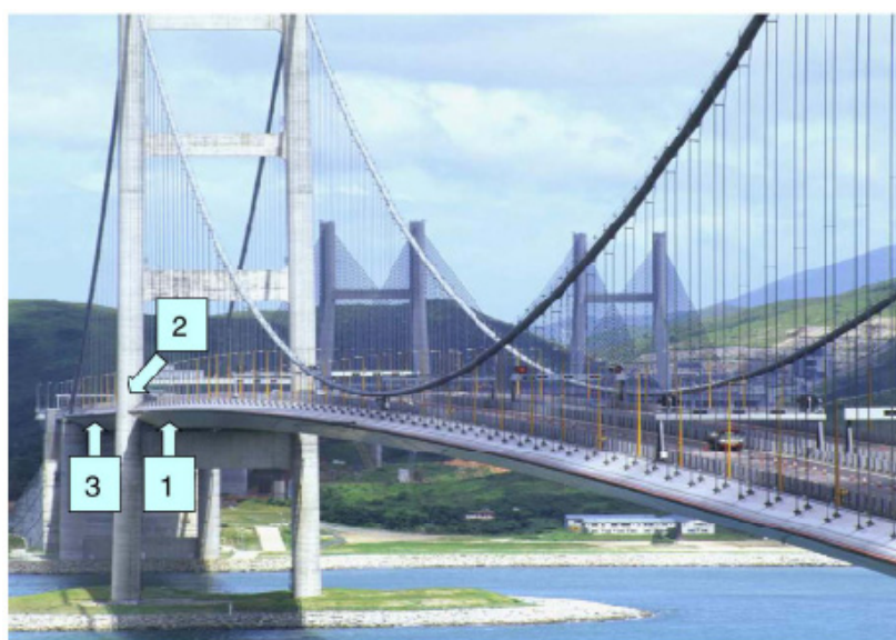
Figure 2. The detail view of FBG sensors installed on (1) hanger cable, (2) rocker bearing, (3) truss girders of section Chainage 23488. Reproduced with permission from [9], copyright 2006, Elsevier.
